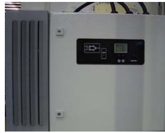
Pictured 500 Ampere 16 kA (Size 800 w x 600 h x 400 d) Wall mounted
